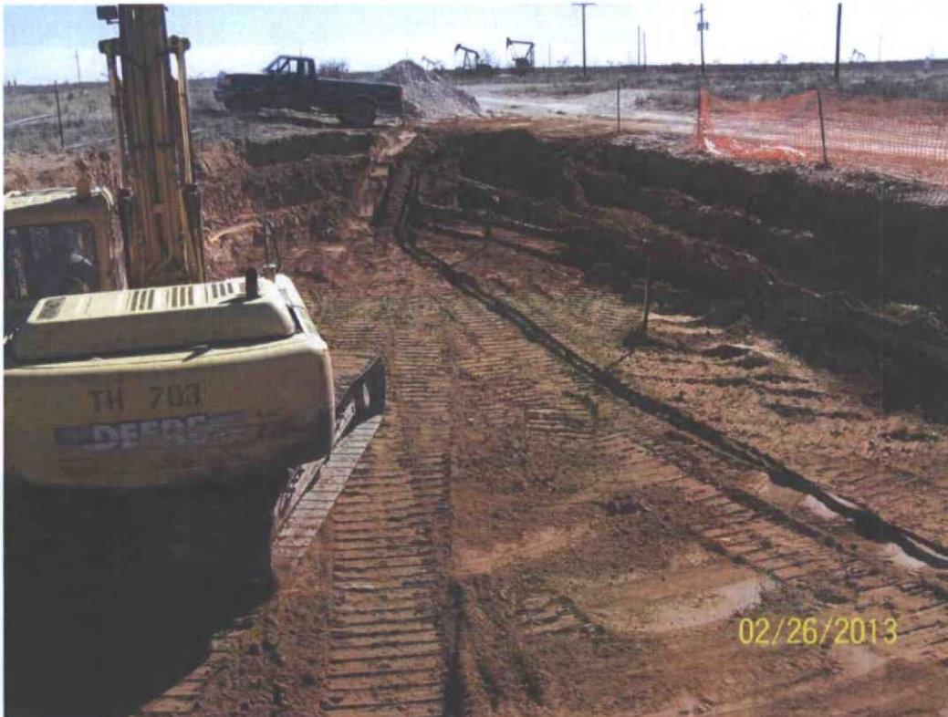
Photograph #7 – Looking southerly at placement and compaction of cushion material layer for placement on 20-mil Polyethylene reinforced liner
