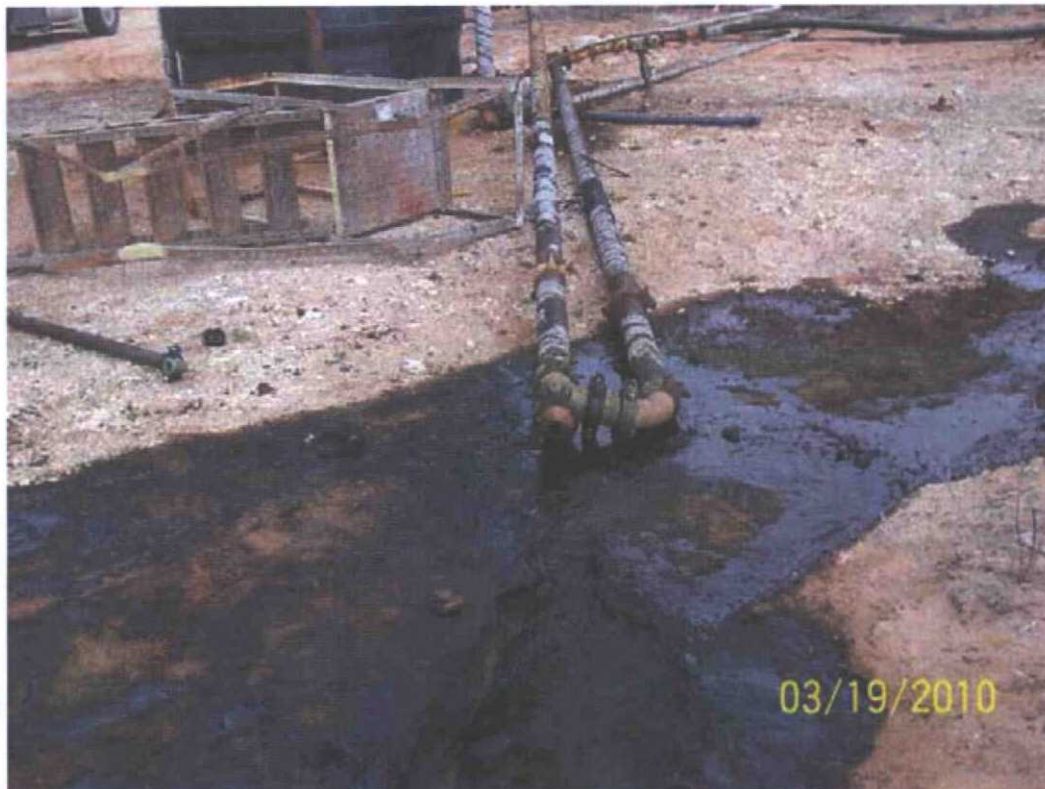
Photograph No. 3 – Looking a broken water leg
