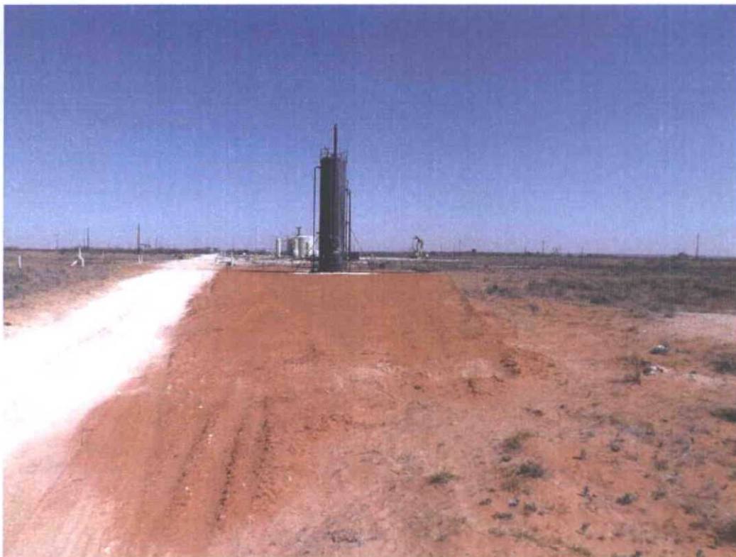
Photograph #10 – Looking northerly at surface of backfilled area and caliche material around heater treater
