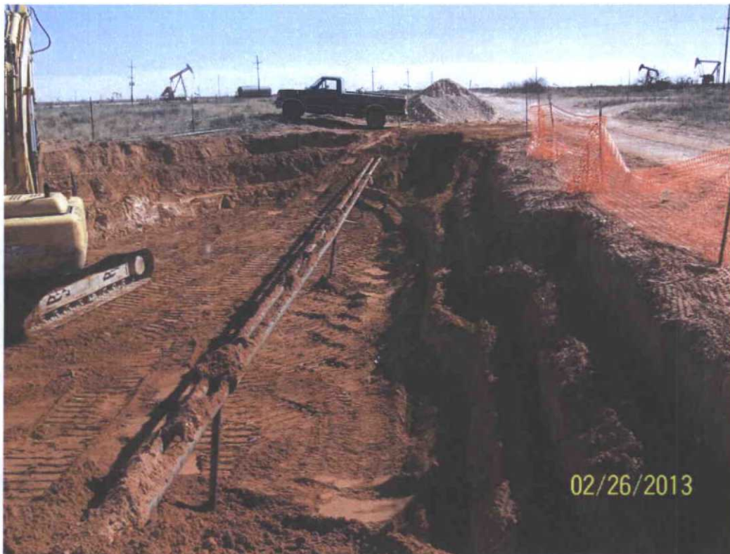
Photograph #6 – Looking southerly at two (2) three-inch steel pipelines with pipe supports and compaction of cushion material layer
