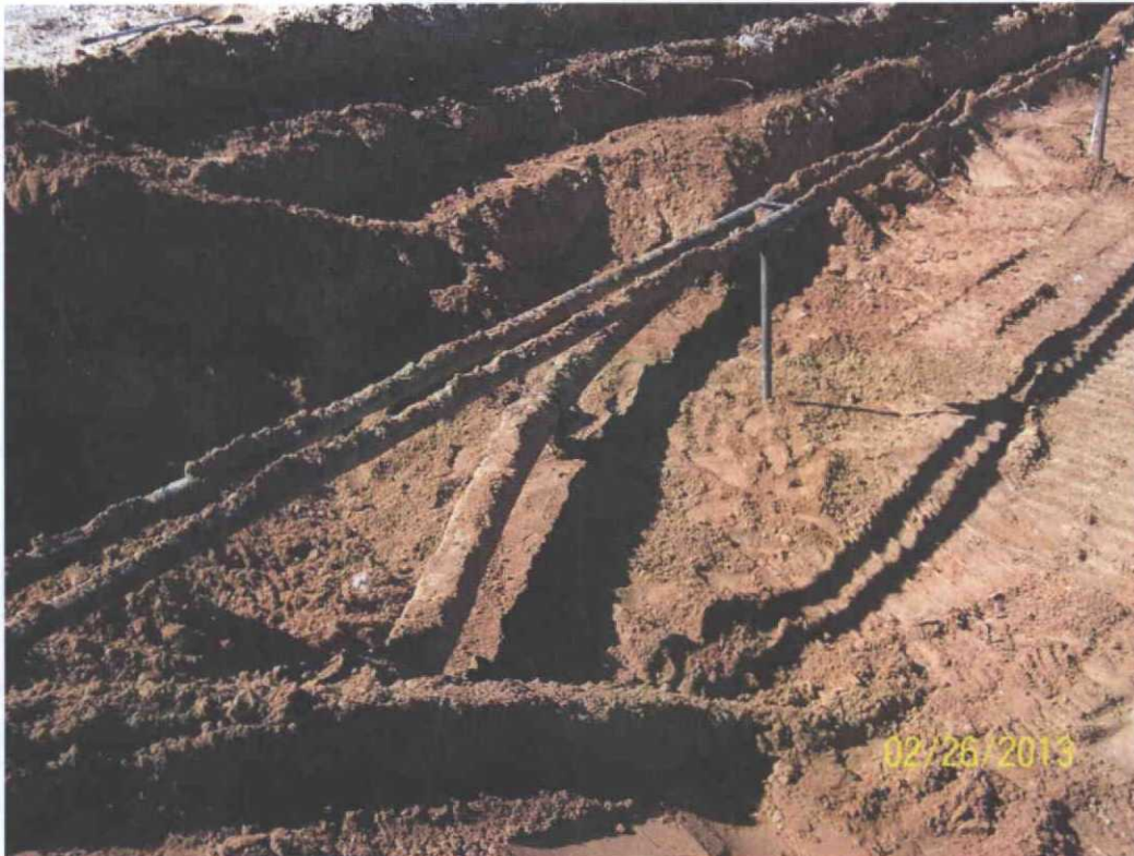
Photograph #5 – Looking at intersection of two (2) three-inch steel and 8-inch poly pipelines
