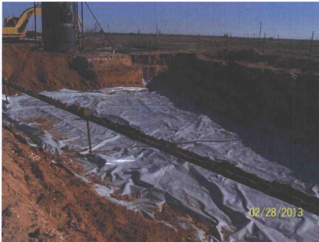
Photograph #8 – Placement of 20-mil Polyethylene reinforced liner
