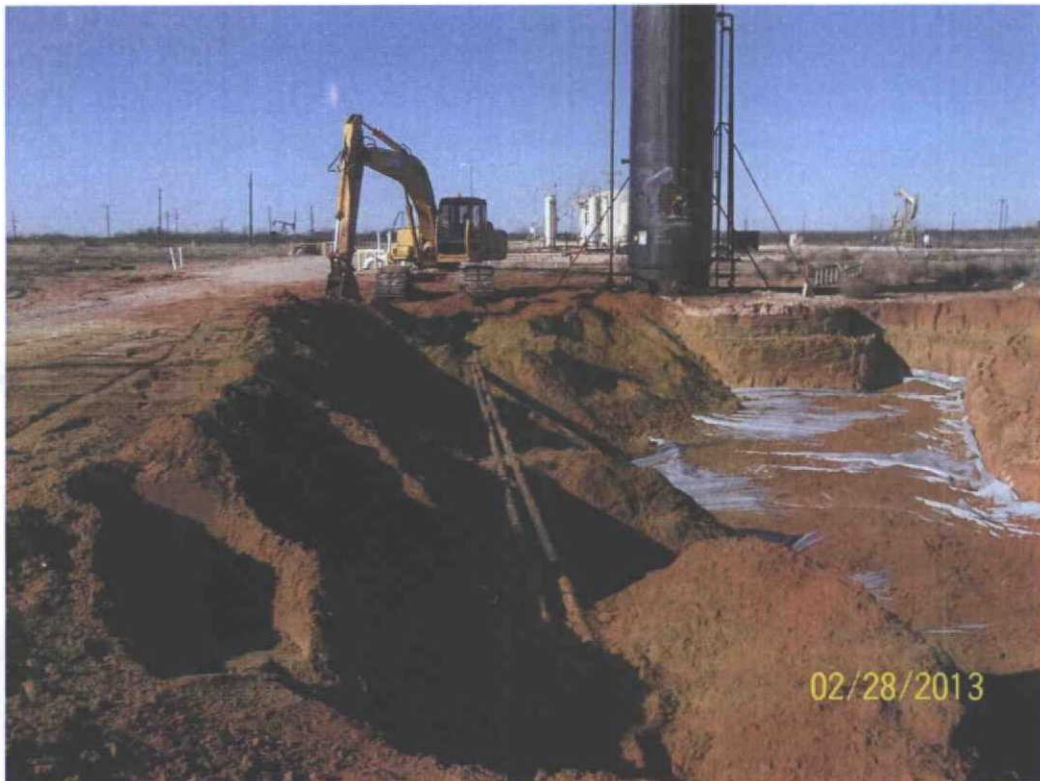
Photograph #9 – Looking northerly at placement of top soil over 20-mil Polyethylene Liner
