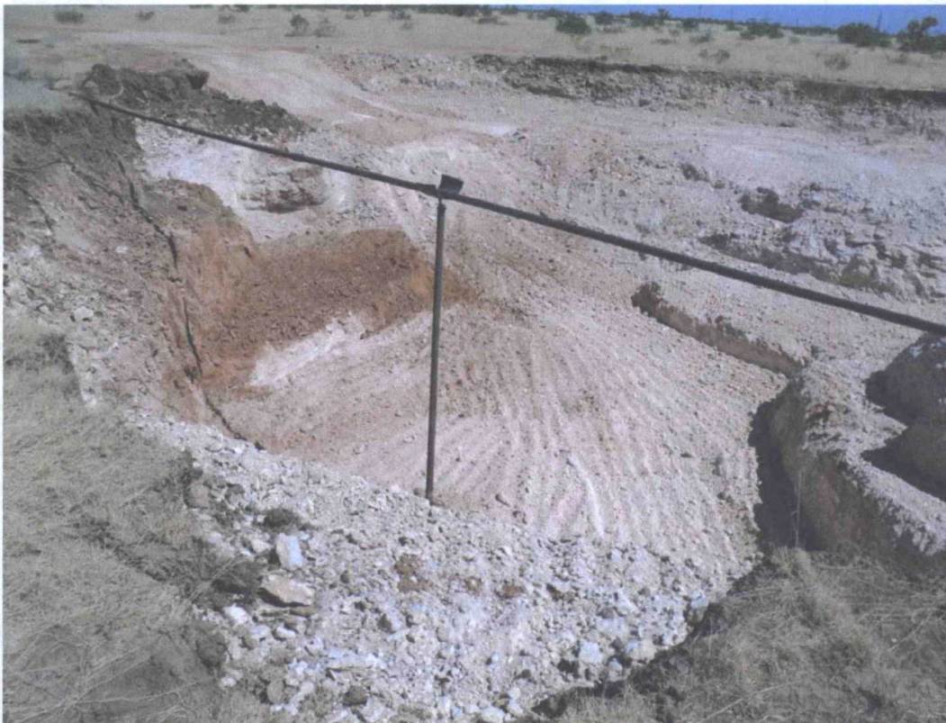
Photograph No. 6 – Looking northerly at excavation, steel pipeline with pipe support and ingress/egress ramp
