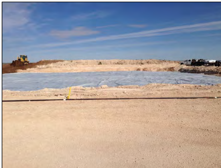
Geomembrane cover installed; backfilling 10/31/2014
