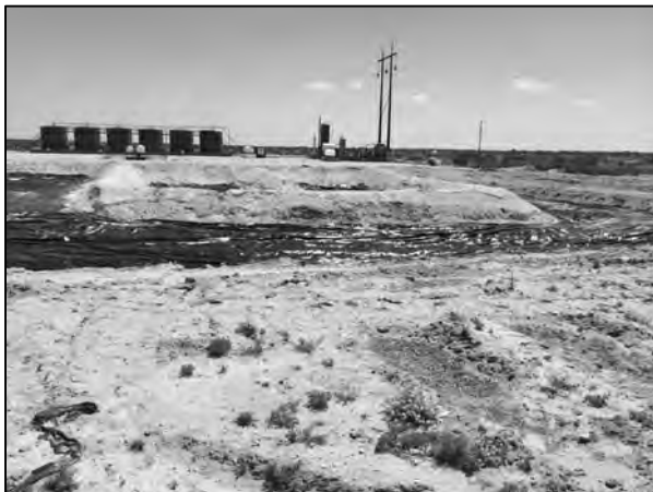
Geomembrane cover over stabilized cuttings 5/8/2015
