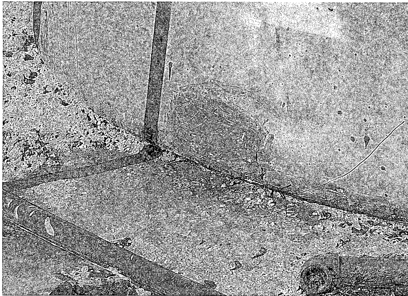
P/W TANK PATCH LEAKING
