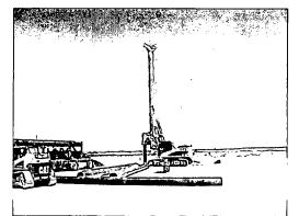
On February 27, 2013 I witnessed the drilling of the rat hole at the Mogi 9 #1H site. Ready Drill LLC of Monahans, Texas performed the work using a track-mounted 30-inch auger drilling rig as shown in the adjacent photograph.
