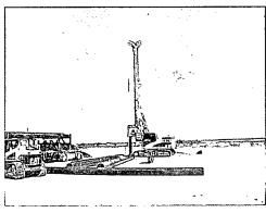
On February 27, 2013 I witnessed the drilling of the rat hole at the Mogi 9 #1H site. Ready Drill LLC of Monahans, Texas performed the work using a track-mounted 30-inch auger drilling rig as shown in the adjacent photograph.
