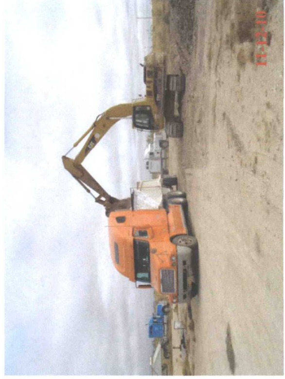
Excavating and loading impacted soil for disposal.
