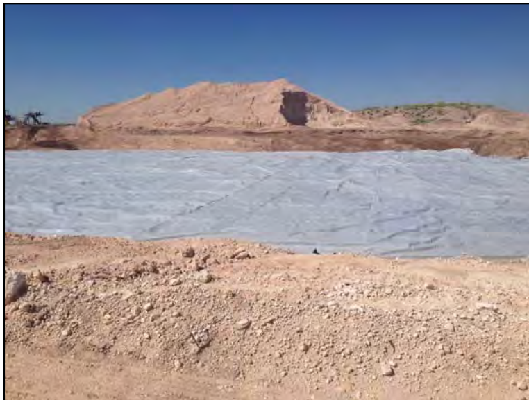
Geomembrane cover installed over stabilized cuttings at 4 + feet BGS 10/9/2014
