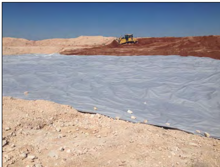
Geomembrane cover installed 10/9/2014
