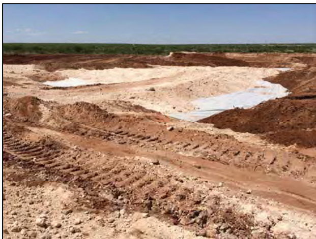
Backfilling over geomembrane cover 5/8/2015
