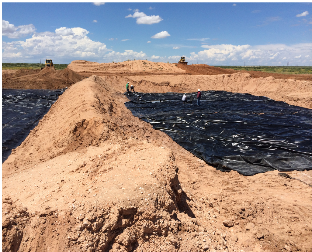
Capping liner photo on 6/10/15
