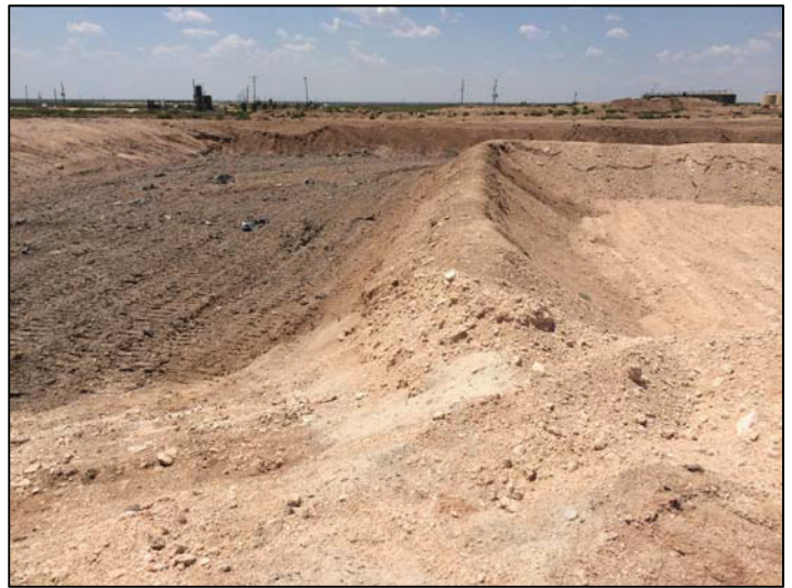
Stabilized cuttings staged for cap liner 8/13/2015
