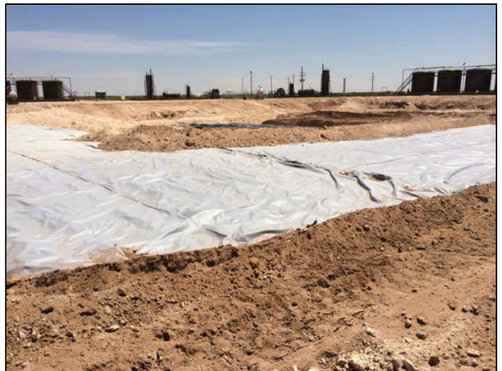
Geomembrane liner over stabilized cuttings 8/18/2015
