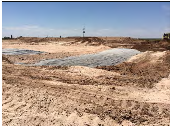
Geomembrane liner over stabilized cuttings 8/18/2015
