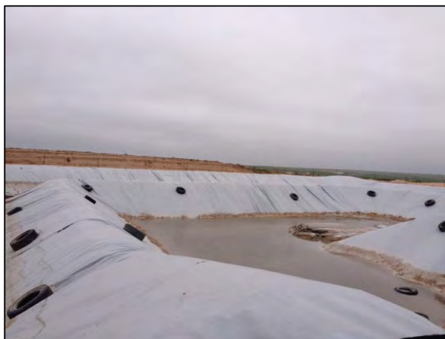
Current liner condition on 5/20/2015; rainwater in pit from previous day
