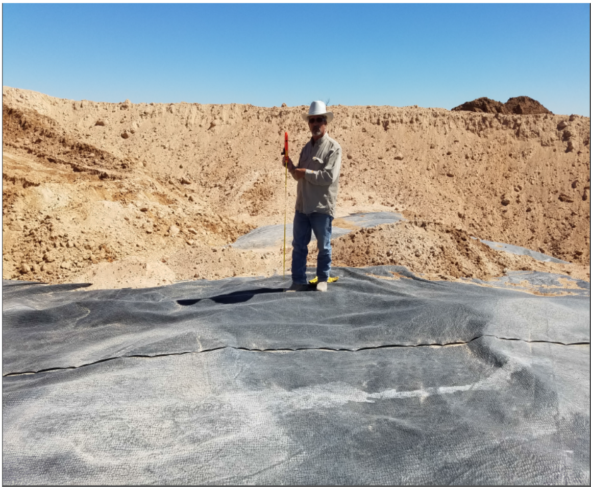
Viewing West 20 Mil. liner installation
