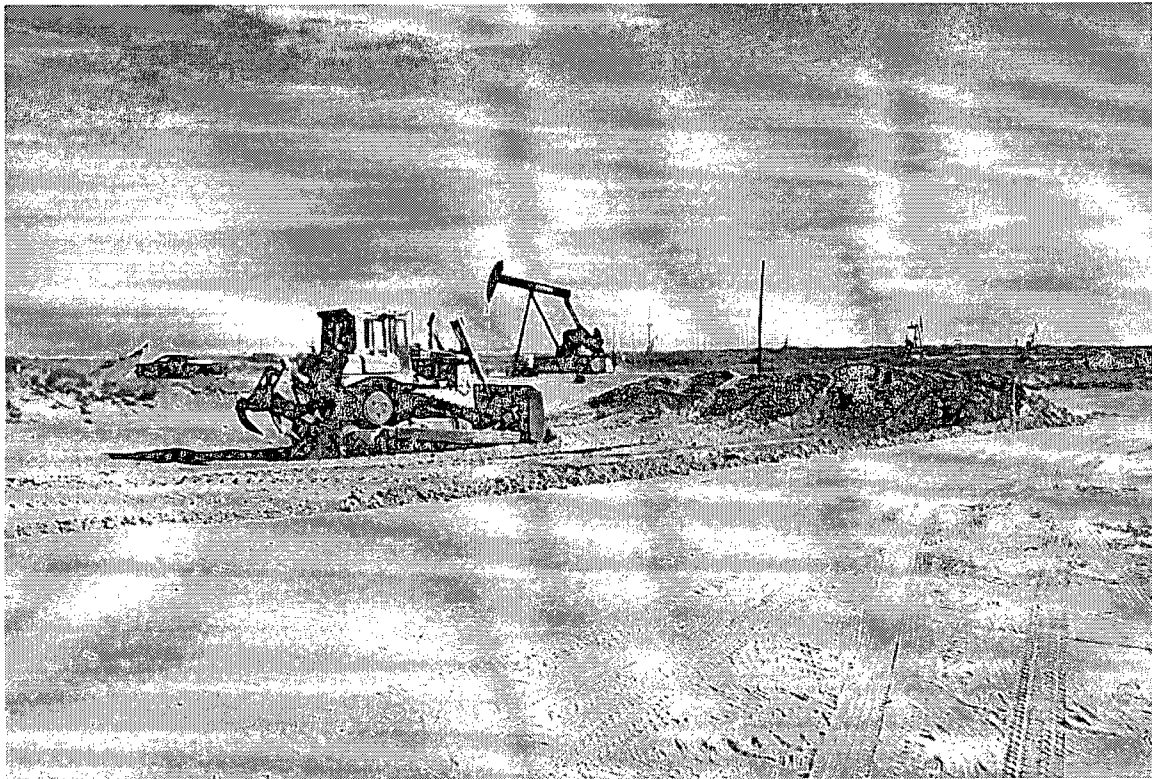
Removing surface caliche layer from the north side of the drill pad
