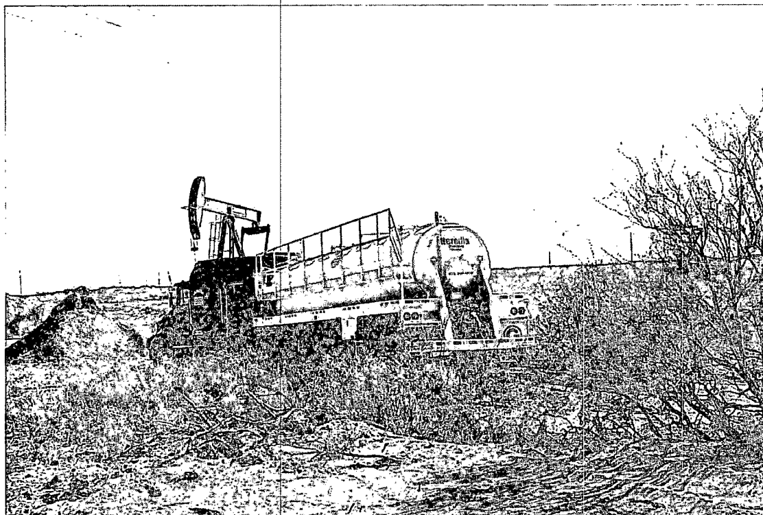
Water truck watering and compacting temporary access along flare fence
