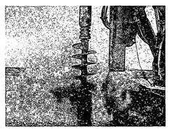
The photograph to the left was taken from the soil recovered at a depth of 98 feet as it is being spun from the auger. This photograph demonstrates the lack of moisture in the cuttings. It is believed that any potential moisture from the bottom or walls of the boring would have been easily identified during the drilling process as each trip into the hole should contact wet soil if it is present at any depth.
