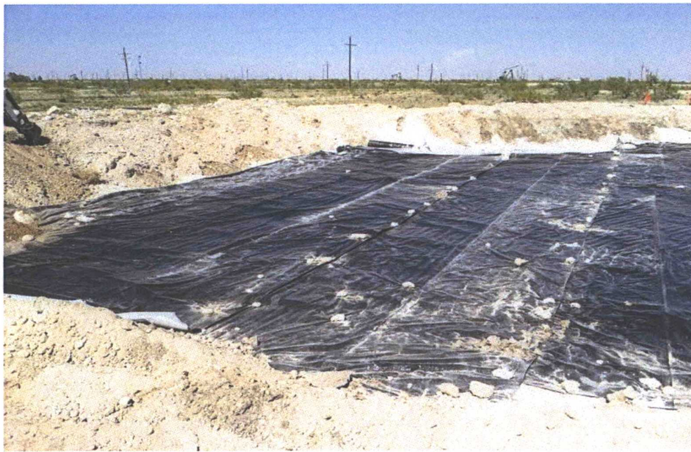
PHOTO 12: View of 20 mil poly liner installation facing northwest
