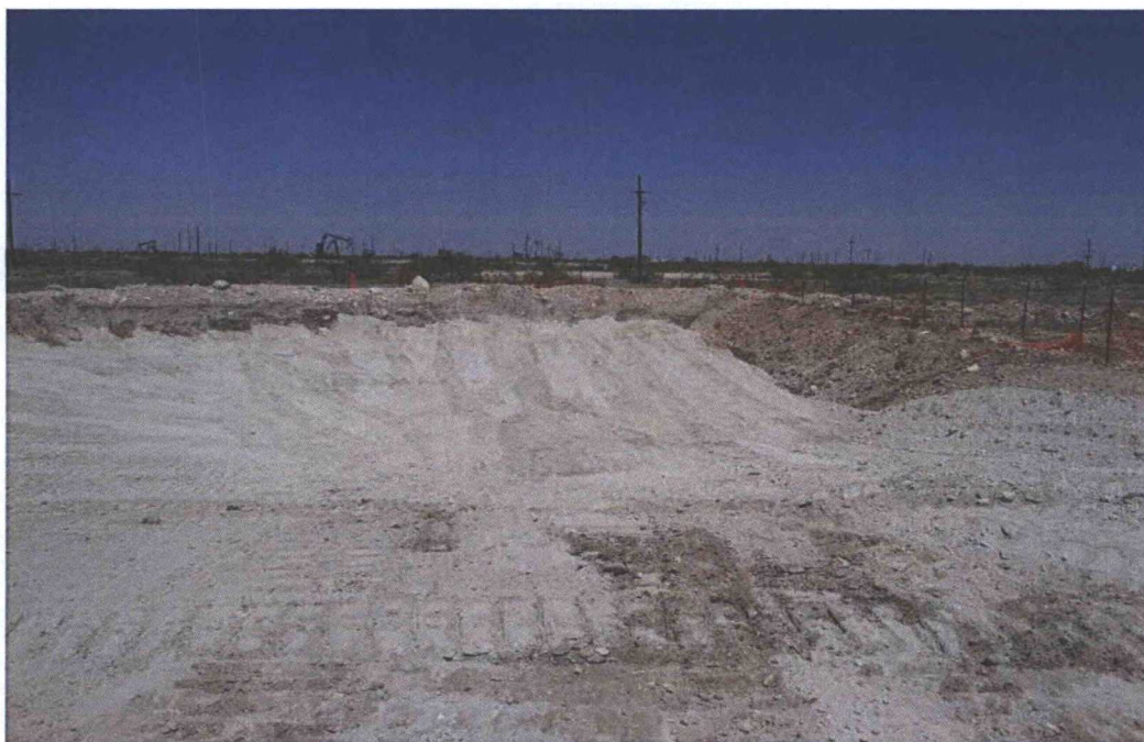
PHOTO 10: View of backfilling activities facing northeast, ready for liner material
