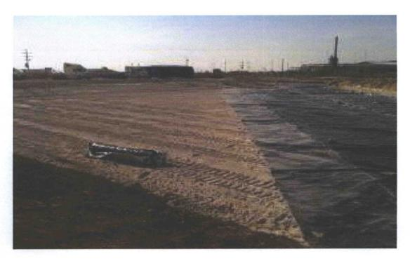
PHOTO 11: View of 20 mil poly liner installation facing southeast
