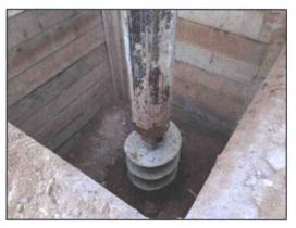
per trip into the hole. I inspected the cuttings from each trip for moisture to indicate a groundwater formation, but all samples were dry. If any appreciable moisture would have been indicated, the operation would have been suspended to allow the water to accumulate and then measured.
