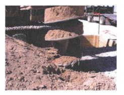
Over the next 2.5 hours the boring was advanced to a total depth of 120 feet by removing approximately 1 to 1.5 feet of material per trip into the hole. Mr. Littlejohn carefully inspected each auger for the appearance of moisture in the soil prior to it being spun off
