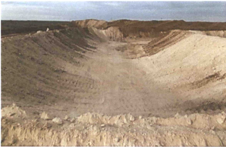
Photograph of suction side of outer horseshoe of drilling cell in Lea County prior to lining.
