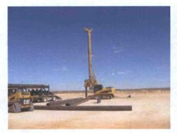
On February 27, 2013 I witnessed the drilling of the rat hole at the Mogi 9 #1H site. Ready Drill LLC of Monahans, Texas performed the work using a track-mounted 30-inch auger drilling rig as shown in the adjacent photograph.
