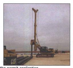
On March 3<sup>rd</sup> and 4<sup>th</sup>, 2014 I witnessed the drilling of the conductor hole for the Bettis 20 State Com 2H well, located in eastern Lea County. Ready Drill LLC of Monahans, Texas performed the work using a track-mounted 30-inch auger drilling rig as shown in the photograph above.
