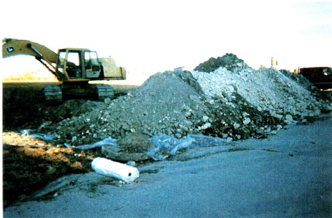
Photo 4: Excavated soil stockpile. View to the east.
