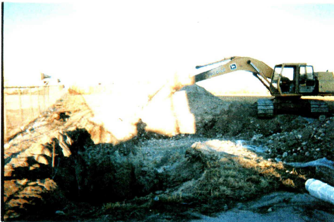
Photo 3: Excavated area of the former oil/water separator and shallow well. View to the northeast.
