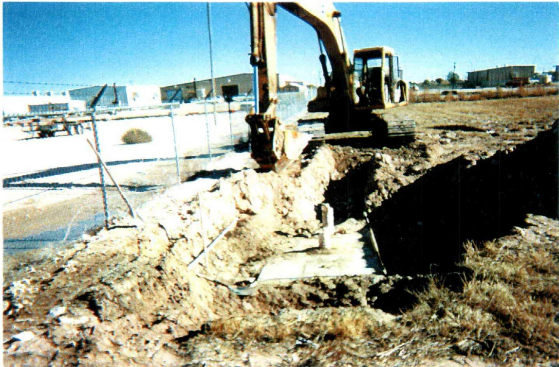
Photo 1: Inactive oil/water separator. View to the northeast.
