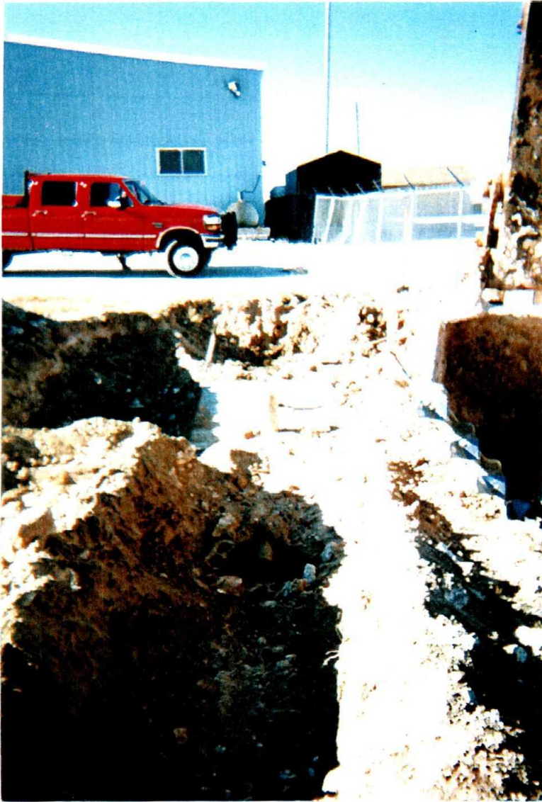
Photo 2: Inactive oil/water separator and shallow well. View to the southwest.
