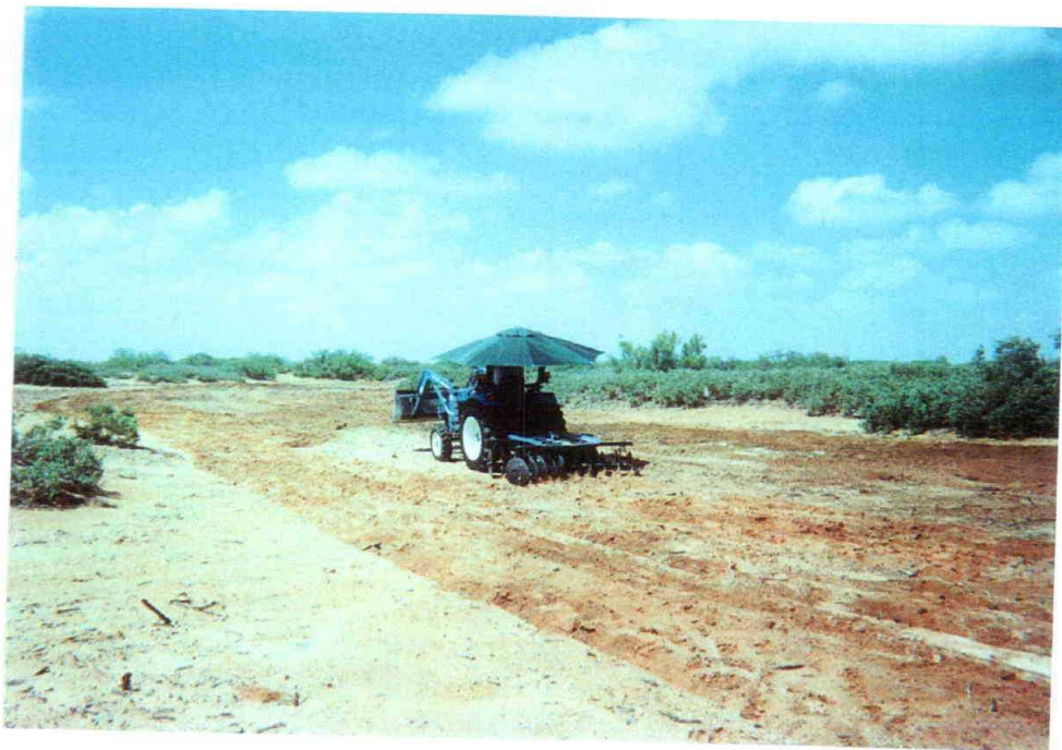
Photo 6: Tilling/seeding of soils along central section of property.
