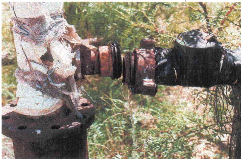
Figure 3: Photograph showing water from storage tank flowing past check valve toward windmill well
