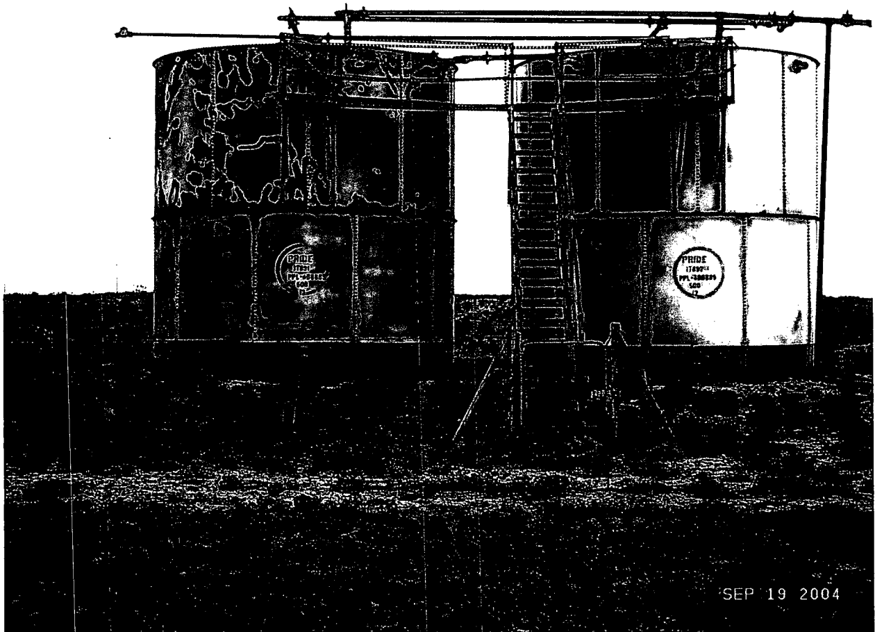
Figure 3. Two 500-barrel Bolted Steel Tanks With Catwalk.
