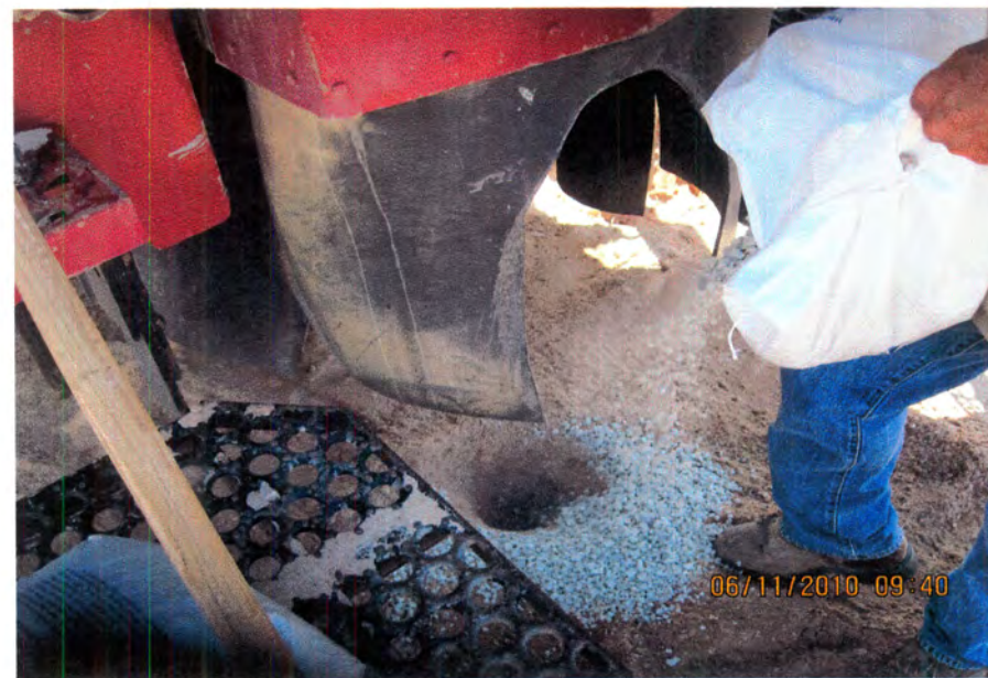
Soil bore # 1 plugged with bentonite
