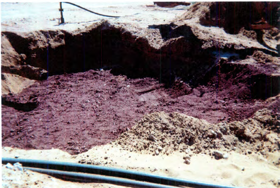
Clay liner installed
