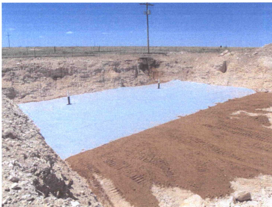
Hahn State Well #1 Release Site - Liner Installation
