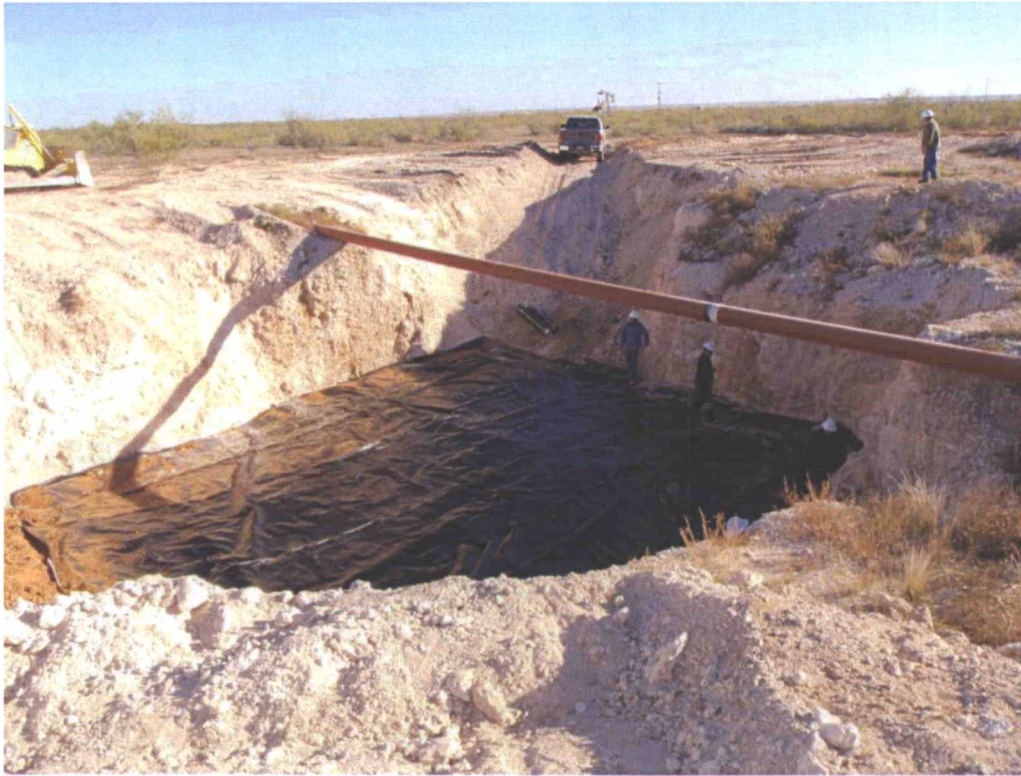
Photograph of the polyurethane liner installation at the A-7 Bettis Release Site.
