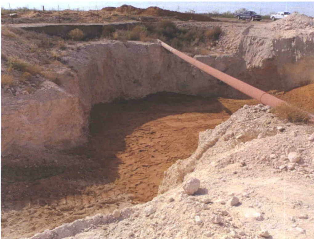
Photograph of backfilling activities and the pad sand installation at the A-7 Bettis Release Site.
