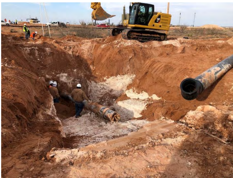
Image 2 – Pipeline excavation occurring .4 miles east of the Longhorn Recycling Facility showing the contact between the caliche and overlying sand.
