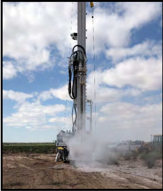
Image 1 - Drilling through dry gypsiferous soils.
