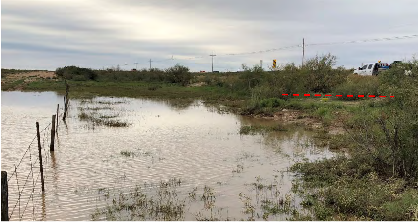
Figure 7 – The warning sign on the highway is above the culvert. The lowest elevation of the culvert appears to be the same elevation as the bench below the dashed red line.
