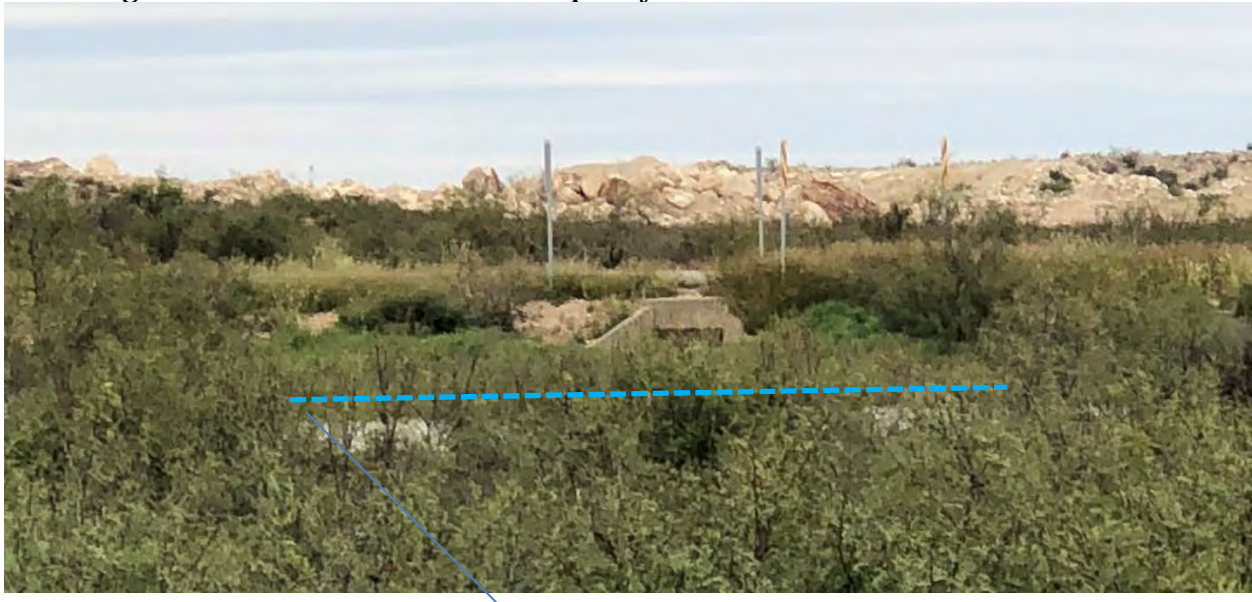
Figure 6 – The culvert beneath the highway will drain water into a mapped watercourse on the east side of the highway. Note that the water level (dashed blue line) appears below the culvert. Signage on the highway is obvious behind the culvert. The rocks in the background are associated with the quarry.
