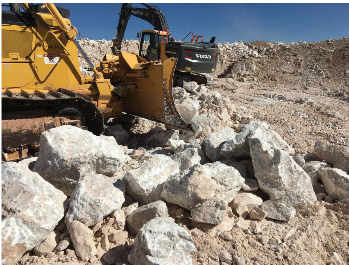
Figure 1: Ongoing Excavation of Floor of South Containment
