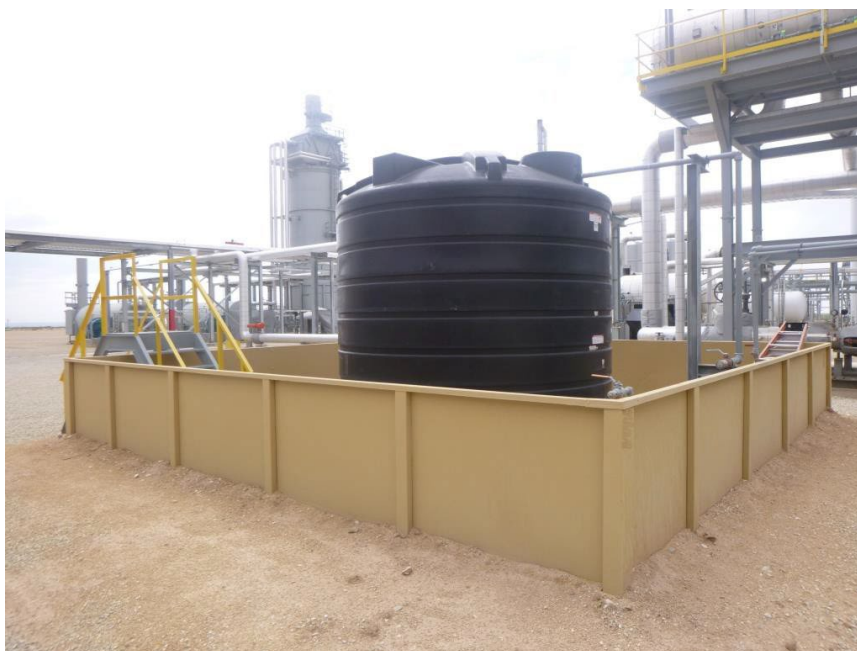
View of Main Containment 3 with metal dike containment, facing west.
