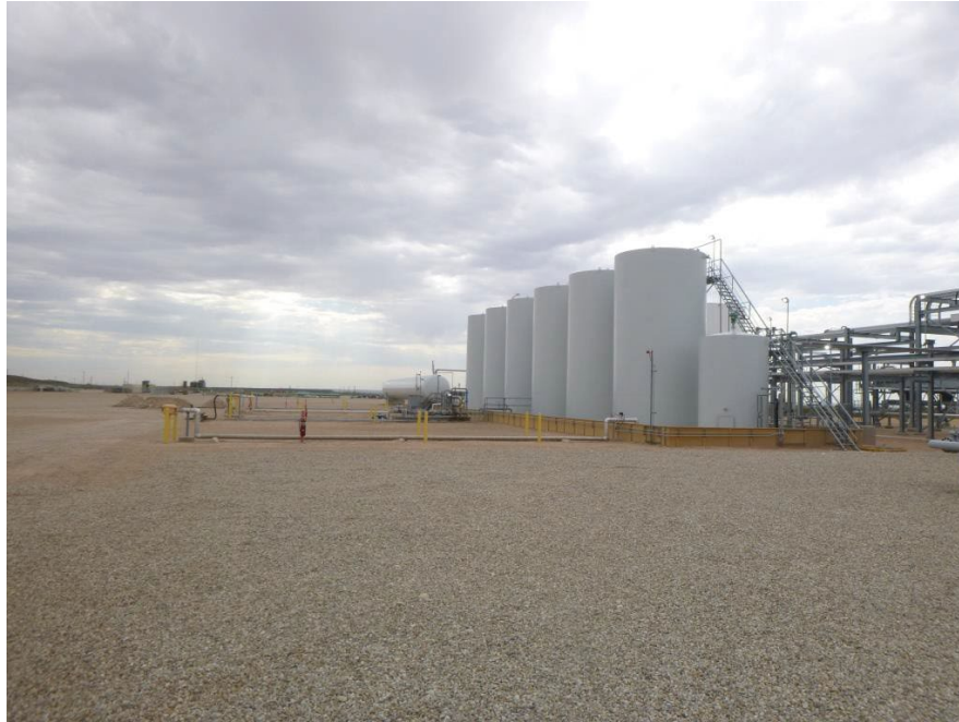
View of Main Containment 1 with metal dike containment, facing south.
