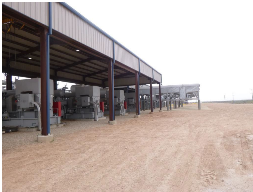
View of the western perimeter of the facility, facing south.
