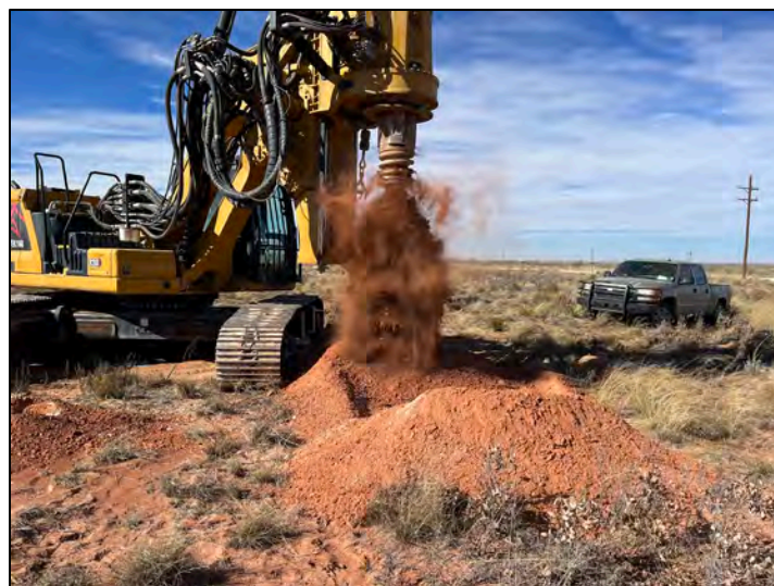
Final TOOH at TD (75 ft); dusty-dry cuttings
