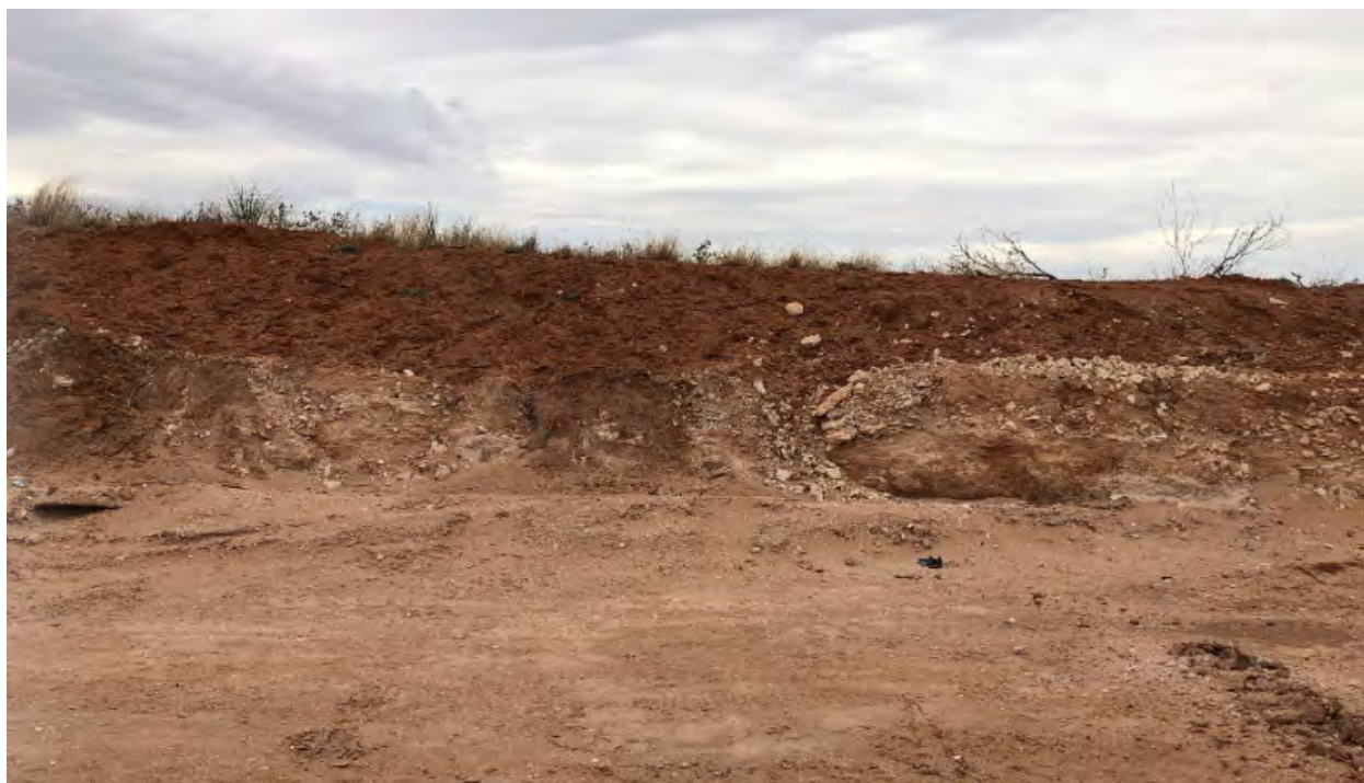
Figure 9 - Exposed caliche in cut wall of westernmost pad.
