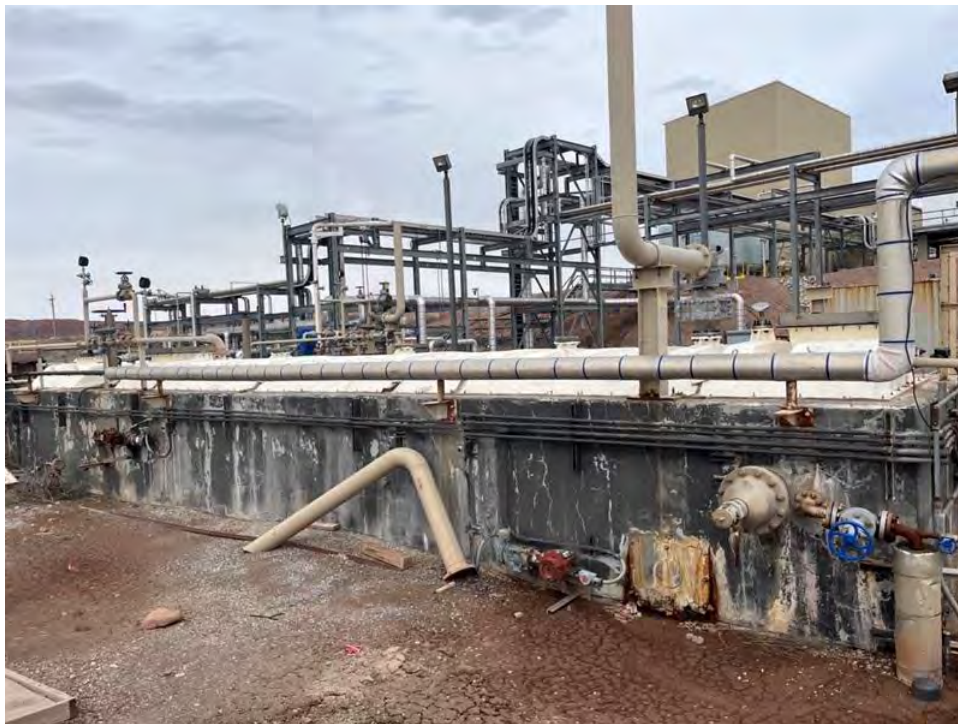
Photo 20. AOC 15 – New API Separator
