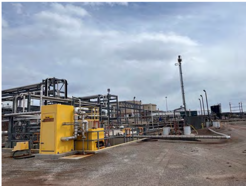
Photo 21. AOC 16 – New API Separator Overflow Tanks
