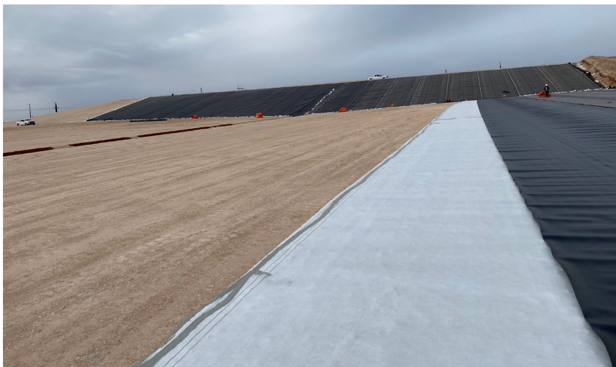
2022-11-16: GCL and FML Deployment
