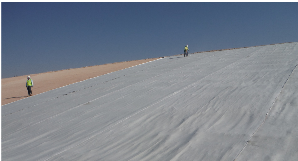
2022-11-15: GCL deployed on the slope
