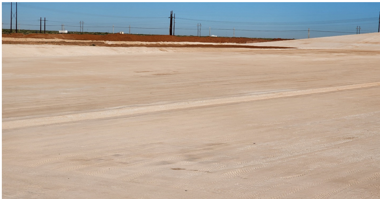
2022-10-11: Completed Subgrade
