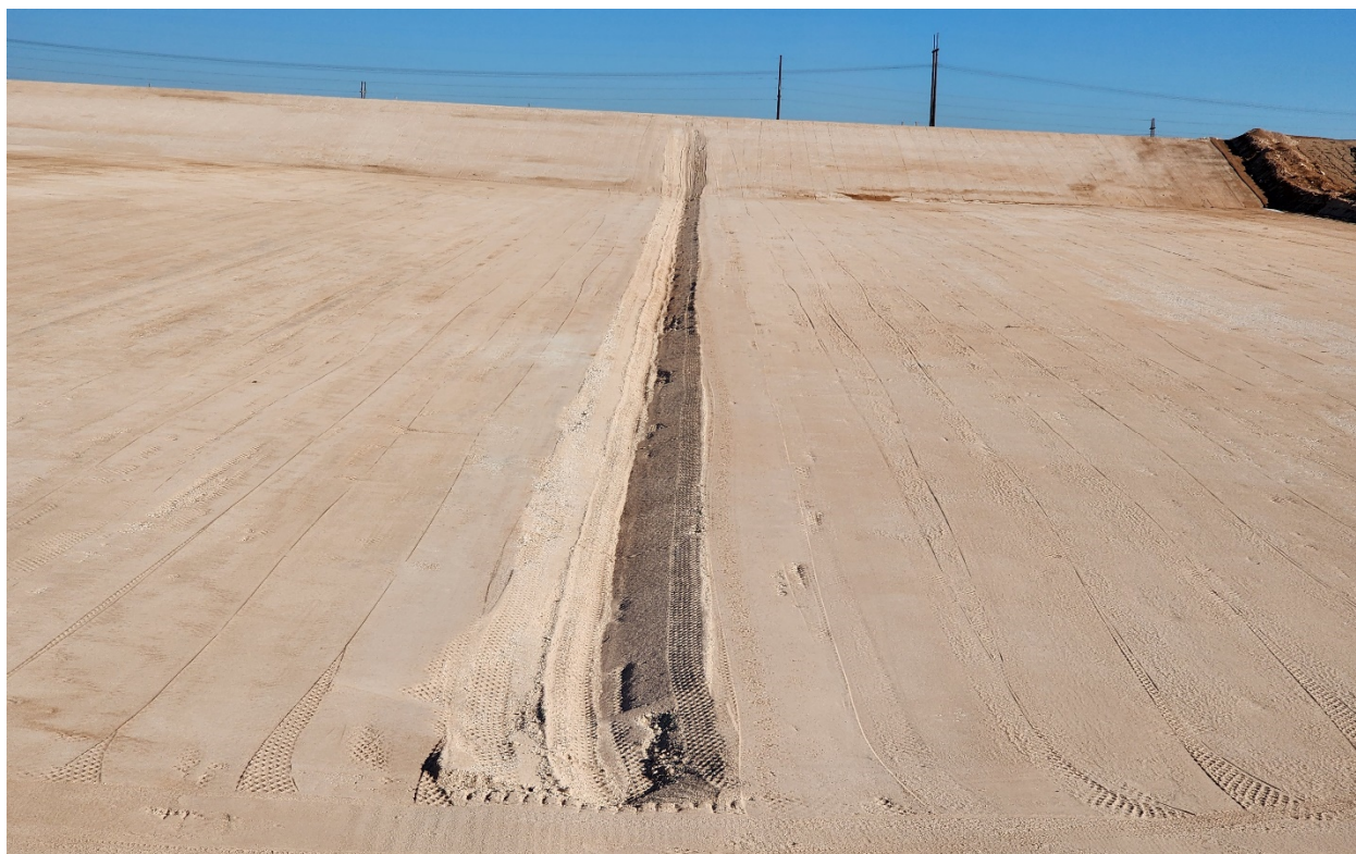
2022-10-11: Completed Leachate Trench
