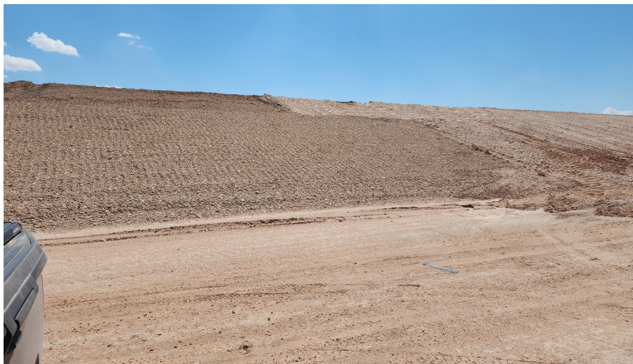
2022-09-15: Side Slope Berm Construction
