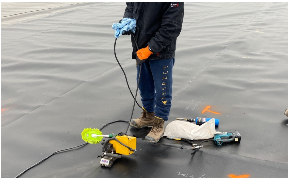
2022-11-16: FML Welding Operations
