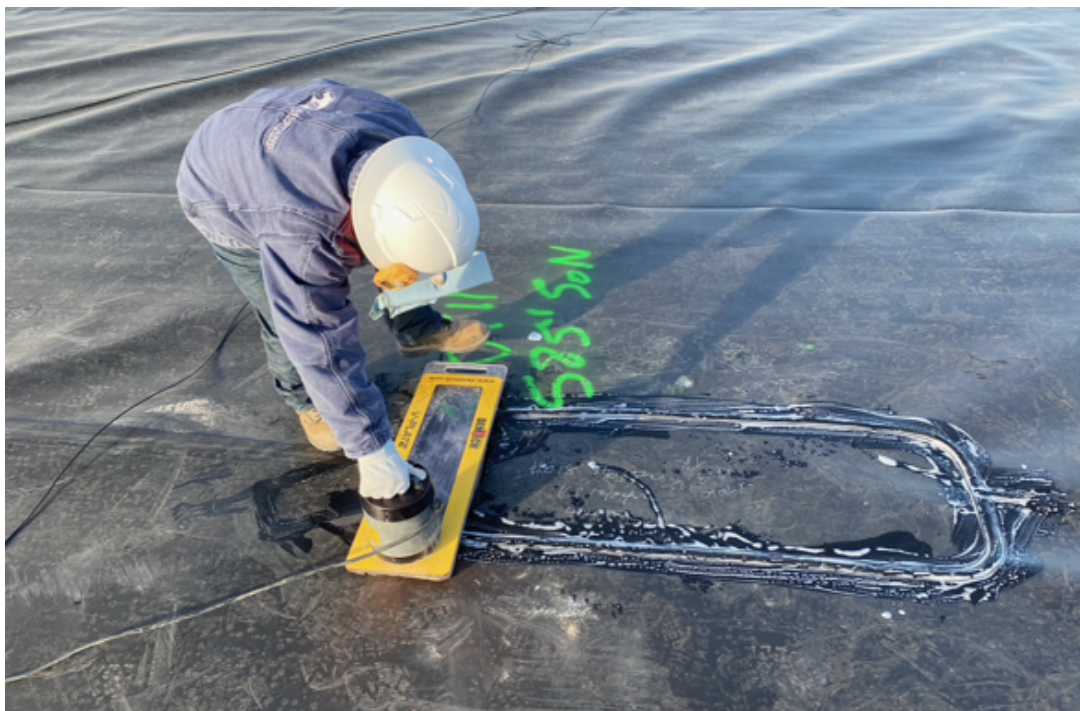
2022-12-05: Nondestructive Vacuum Testing of Repairs
