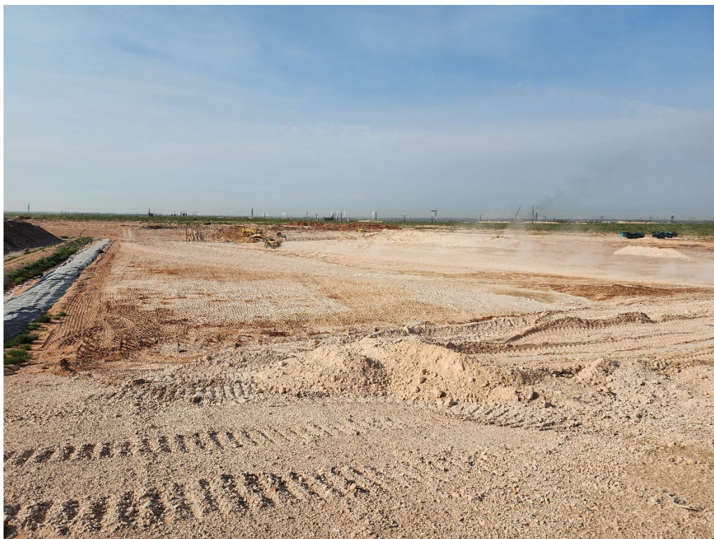
2022-09-09 Excavation of Cell 4AB.
