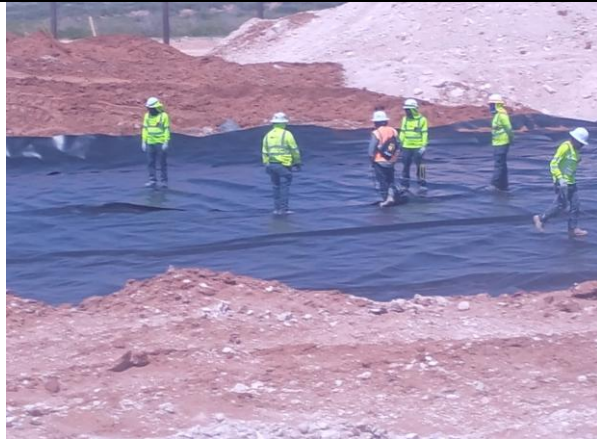
Photo 1: Overview of liner installation.
