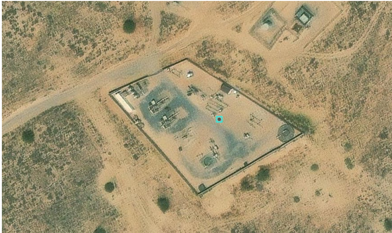
Figure 1.2 Buena Suerte Compressor Station
