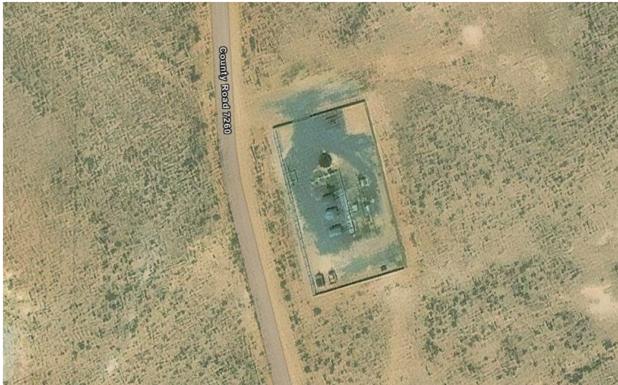
Figure 1.1 Bisti Compressor Station
