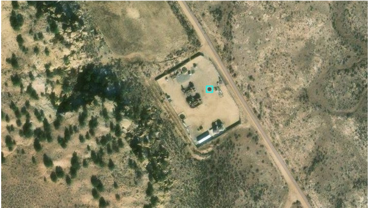
Figure 1.5 Otero Compressor Station
