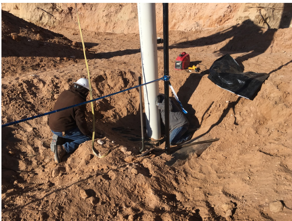
Photo of Installing 10" Casing for BH 1
