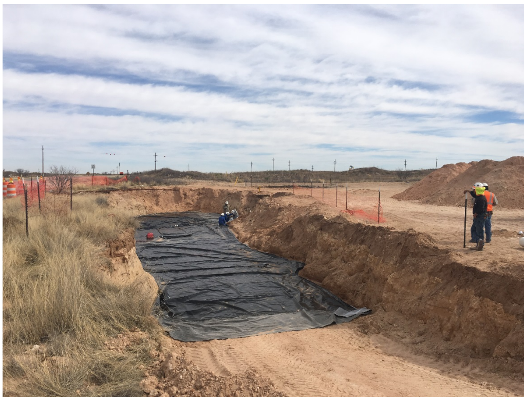
Photo of Sowing New Liner to Existing Liner
