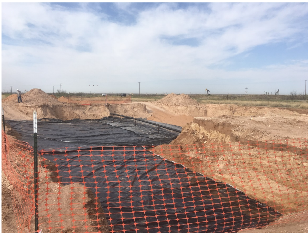
Photo of Liner for South Excavation
