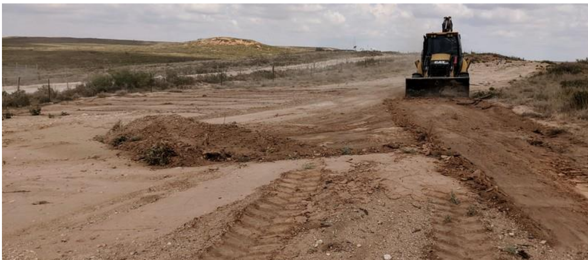
Figure 3: Excavation of source material - hauled off for proper disposal. Photograph is viewing northwest from southeastern release extent. GPS: 32.4513564 N, 103.6196942 W. Date/Time: 2020-09-17 11:24:43
