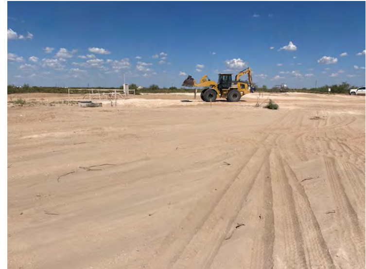
Photograph 12: View of completed backfill.
