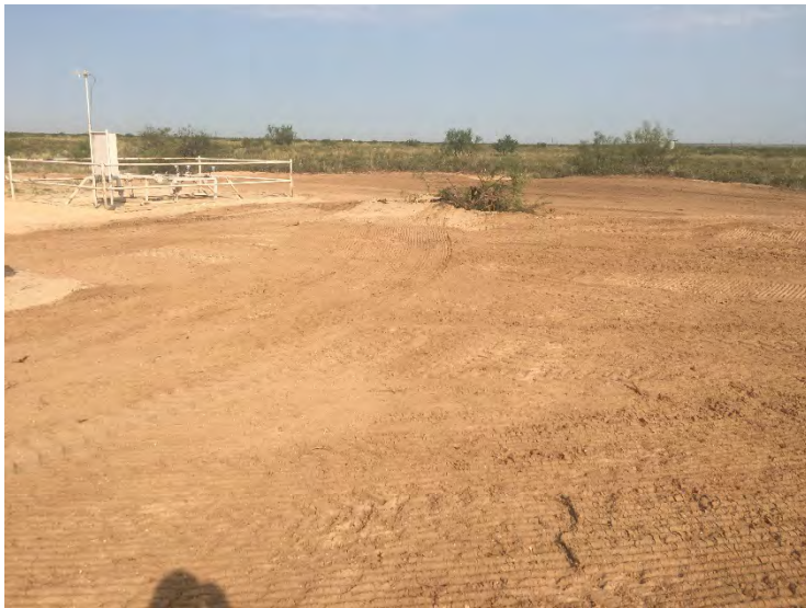
Photograph 15: View of completed re-seeding facing NW
