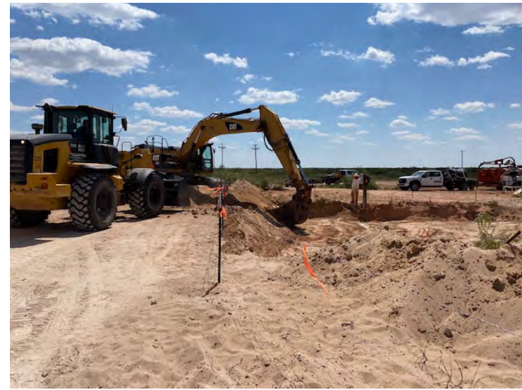
Photograph 4: View of trackhoe excavating in the SE section of the excavation.
