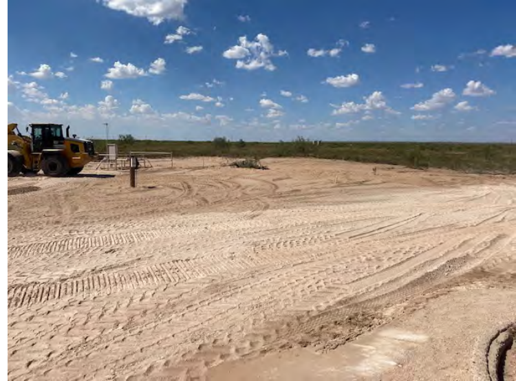
Photograph 14: View of completed backfill and lease road facing NW
