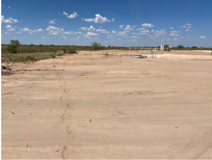
Photograph 13: View of completed backfill facing NE
