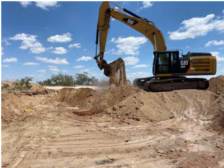
Photograph 3: View of trackhoe excavating in the central section of the excavation facing E.
