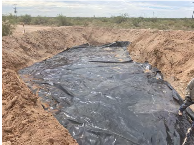
Photograph 11: View of liner installed in SW section of excavation.
