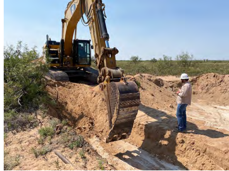
Photograph 2: View of trackhoe excavating in between lines, facing NW
