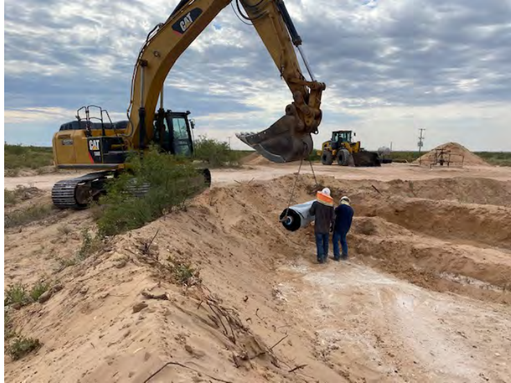
Photograph 9: View of liner installation process starting.
