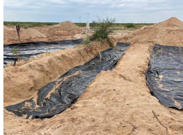
Photograph 10: View of liners installed in the NE section of excavation
