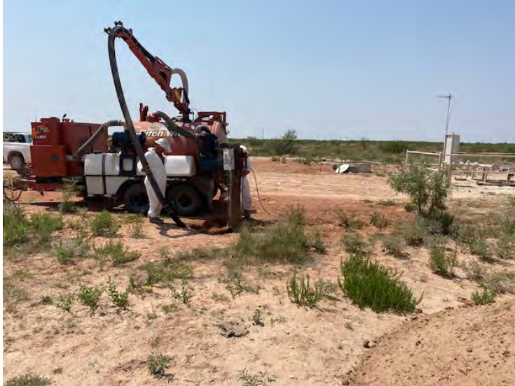
Photograph 1: View of hydrovac exposing electrical lines
