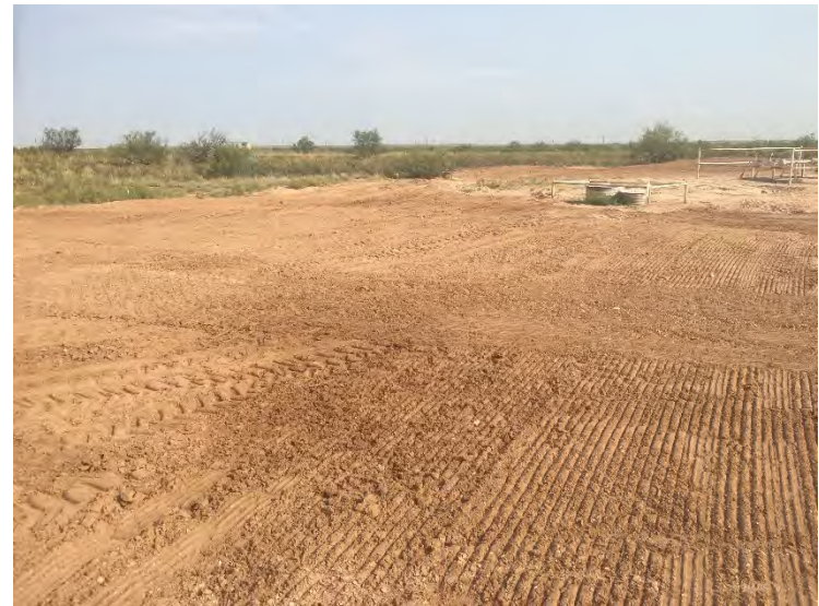
Photograph 16: View of completed re-seeding facing NE
