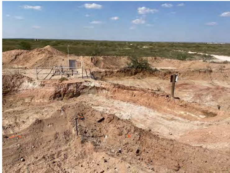
Photograph 7: View of complete excavation, central section, facing N.
