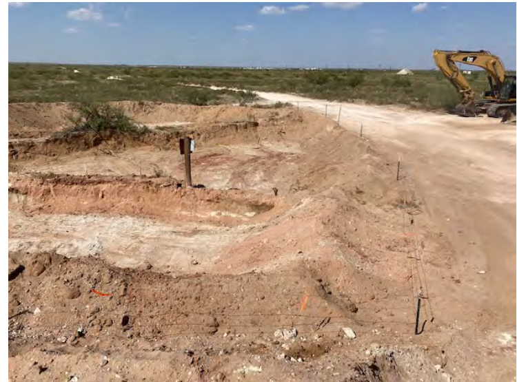
Photograph 8: View of complete excavation, NE section, facing NE.
