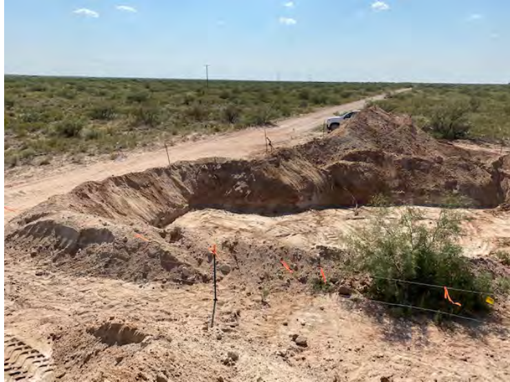
Photograph 5: View of complete excavation, SW section, facing W.
