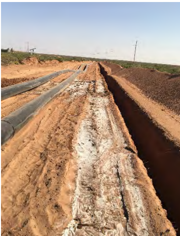
5. View of spill tracking into new pipeline ditch.
