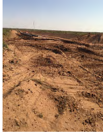
4. View of new pipeline construction in spill path.
