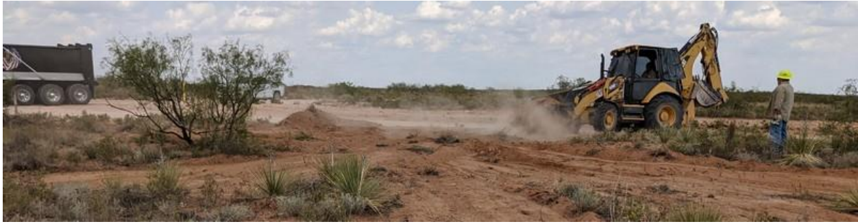
Figure 3: Excavation of source material - hauled off for proper disposal. Photograph is viewing northeast from southwest corner of release extent. GPS: 32.4341378 N, 103.5496806 W. Date/Time: 2020-09-16 13:38:55
