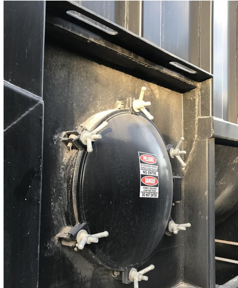
Leak source – tank hatch not fully closed
