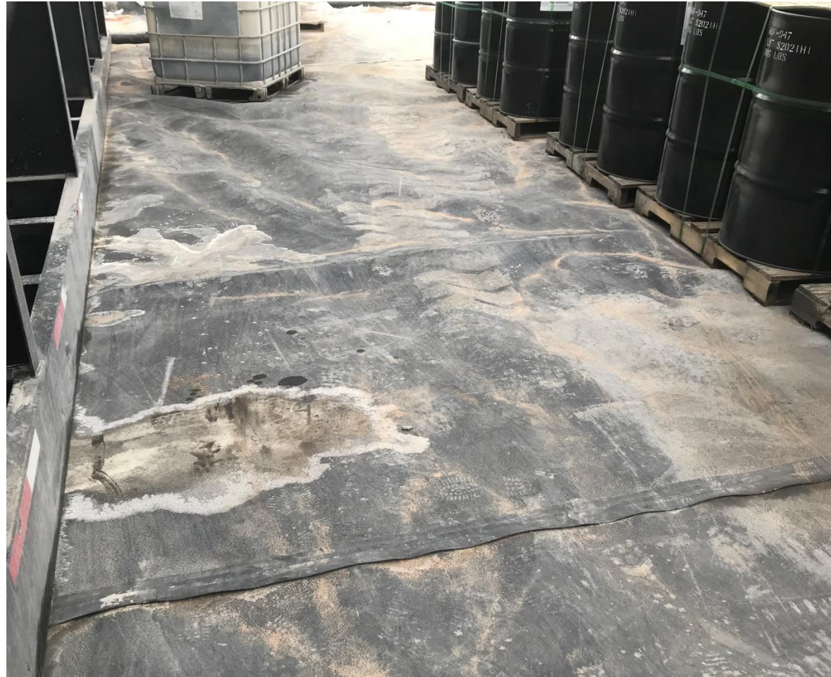
Liner Seam Integrity Appears Intact
