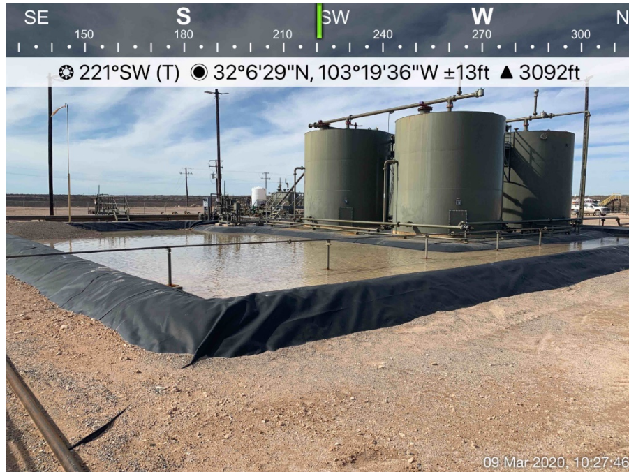
Stormwater contained within lined berm, viewing southwest
