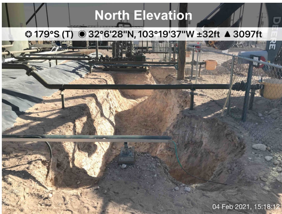
Soil excavated to a depth of 4.1 feet bgs encompassing C-5 and C-6, February 4, 2021
