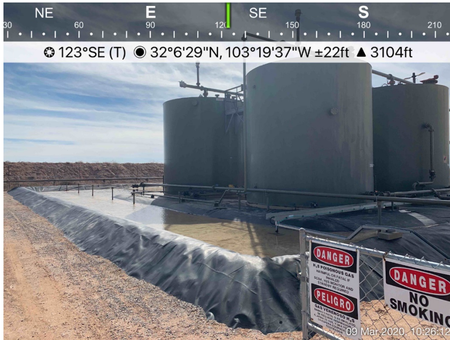
Stormwater contained within lined berm, viewing southeast
