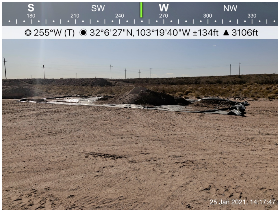
Soil stockpiled on liner prior to removal, January 25, 2021
