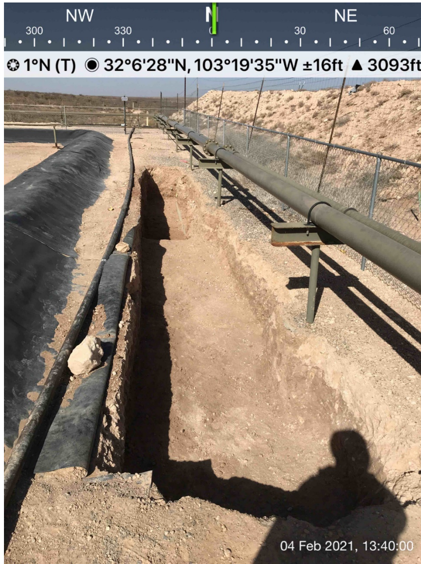
An additional 1 foot excavated from the sidewall of C-4, February 4, 2021
