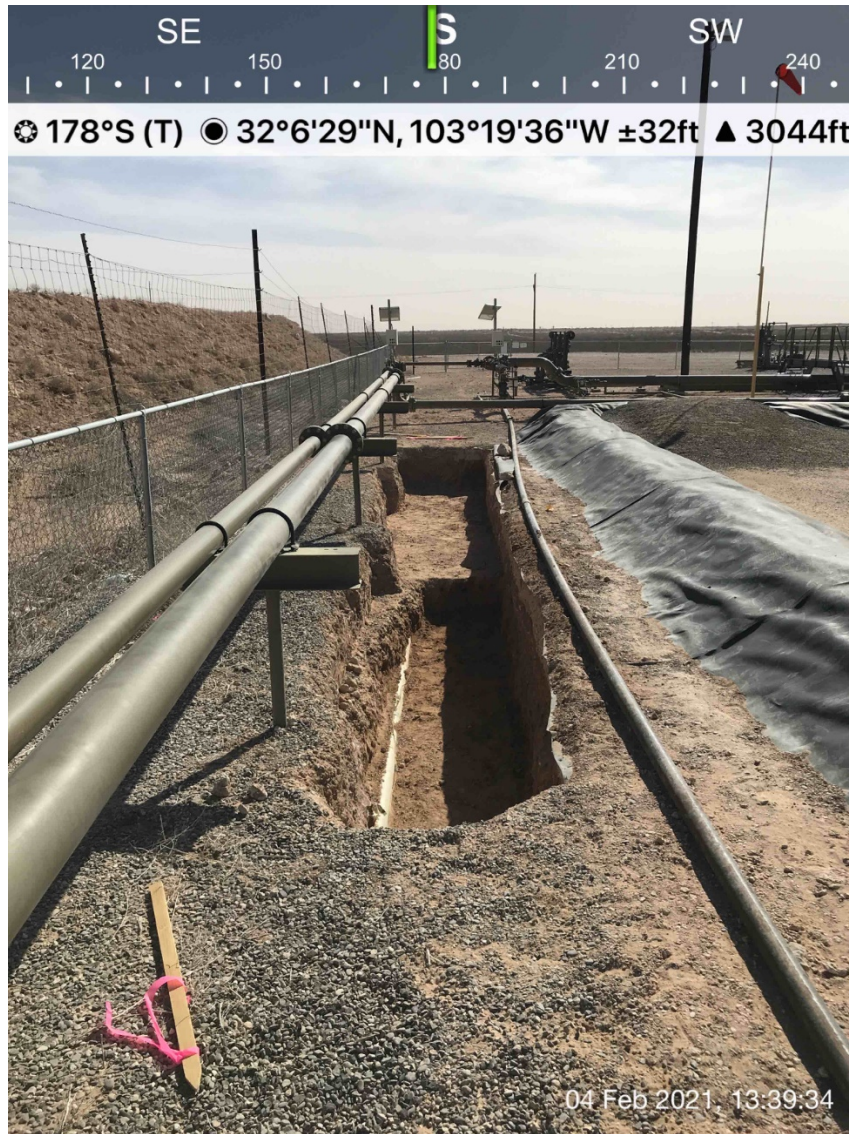
Soil excavated encompassing C-2 to a depth of 3 feet bgs, February 4, 2021
